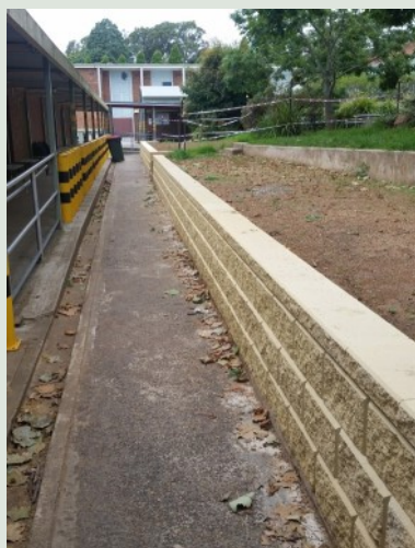
The retaining wall outside D Block has been replaced due to structural and water drainage issues.
